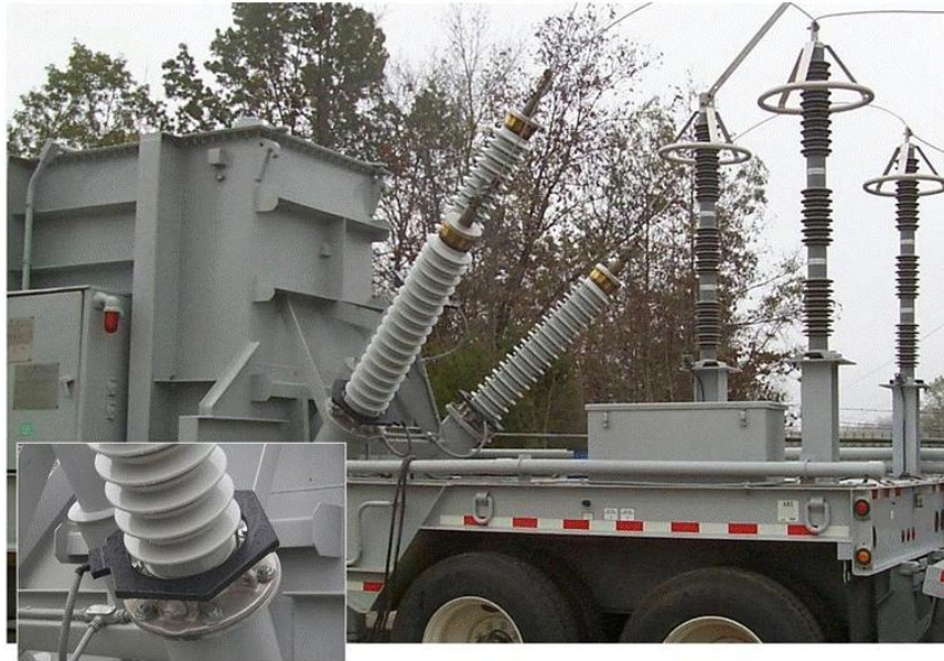
Figure 4-20. Rogowski Coil Installation around Bushings in a Mobile Substation
