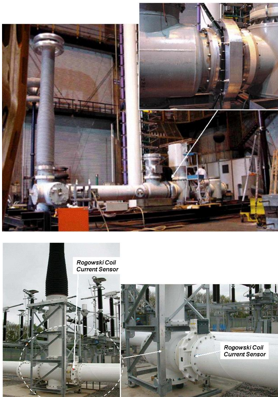
Figure 4-24. Rogowski Coil implementations in GIS (example 3)
